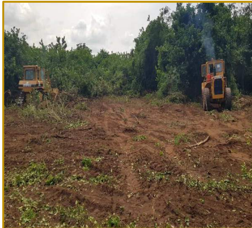
Land being cleared
